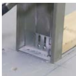
Attach base anchors to floor
